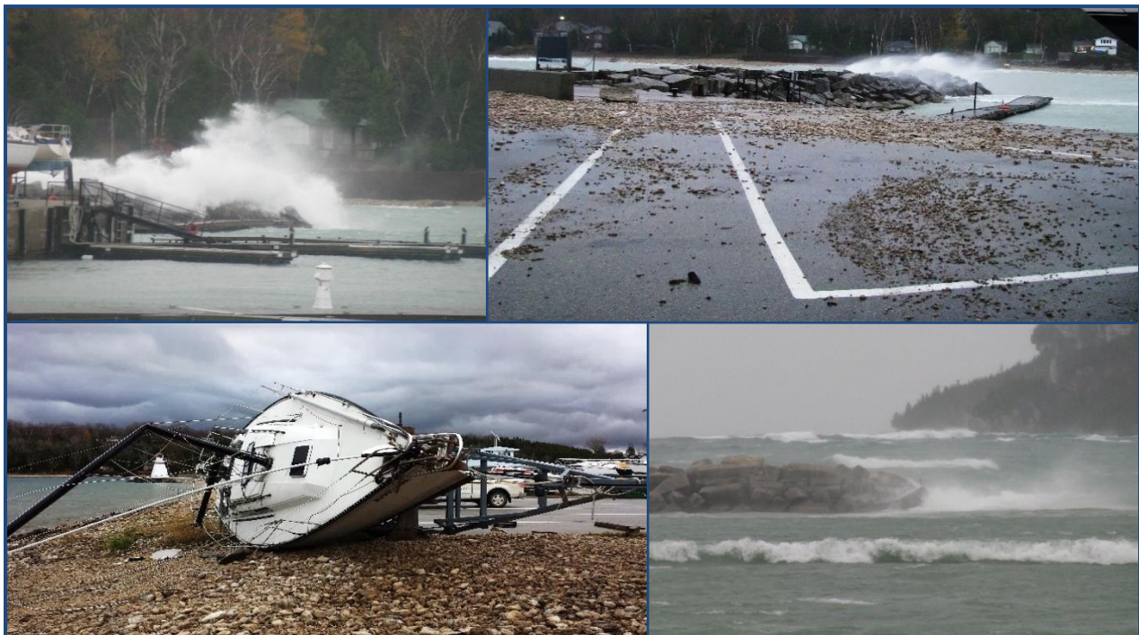
Figure 3-2: Weather and Damage During Storms at Lion's Head Marina
