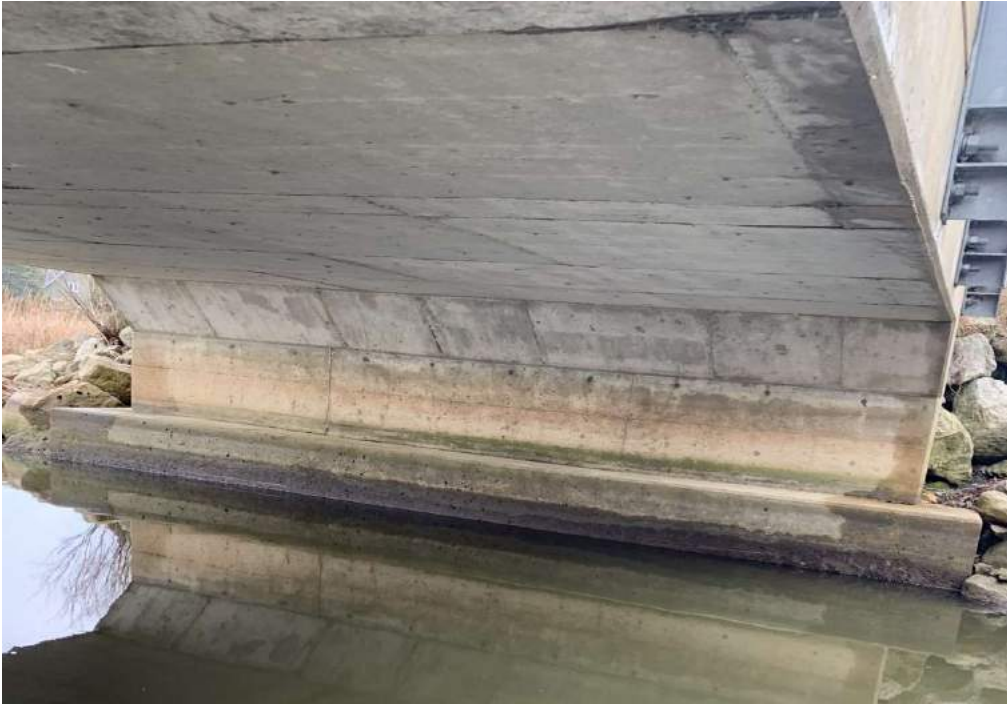
11-4: View of structure soffit
