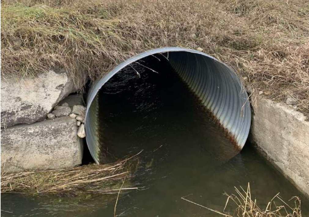
Photo 15-4: View of west culvert end
