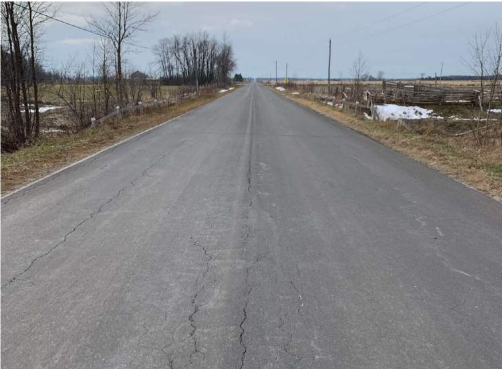
Photo 16-7: View of structure from approach
