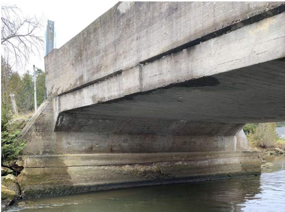
Photo 6-7: View of structure soffit and footing/abutment wall.
