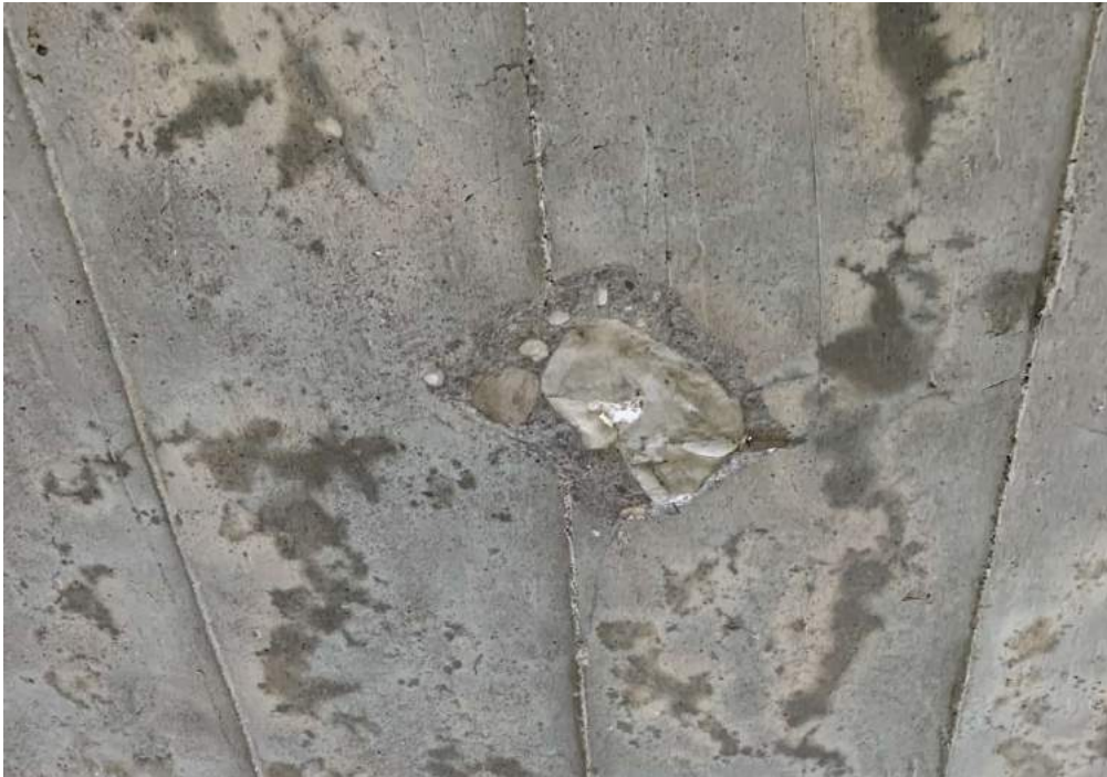
Photo 8-10: View of structure soffit
