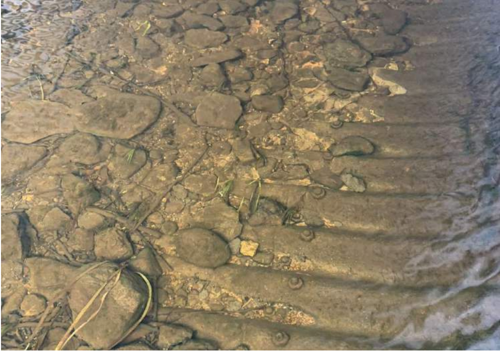
Photo 14-6: View of culvert barrel interior
