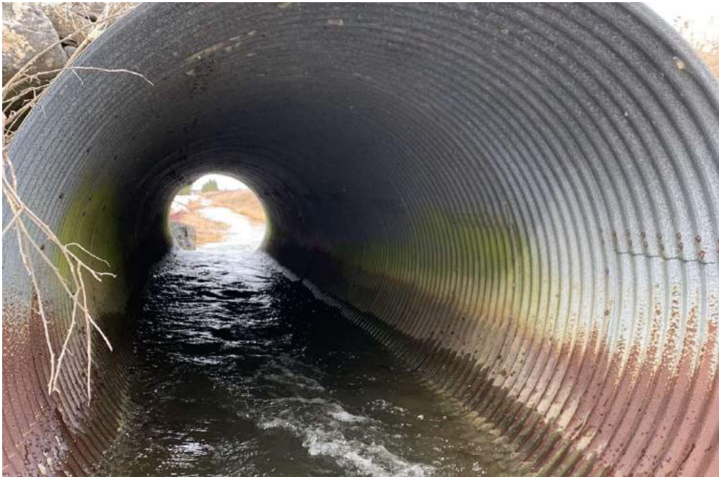
Photo 18-9: View of west culvert barrel interior
