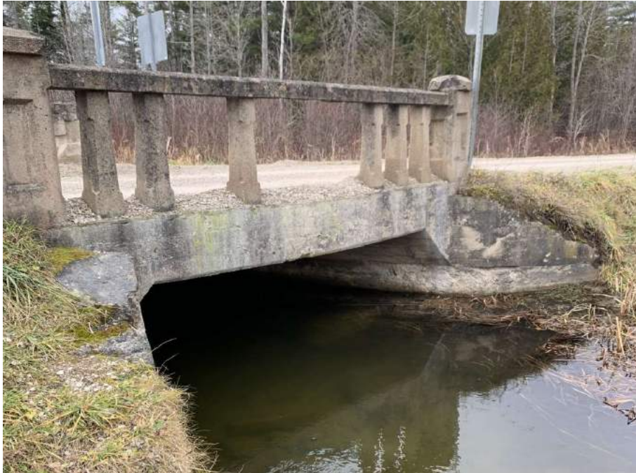
Photo 4-2: View of east structure elevation, wingwalls, exterior curb and barrier
