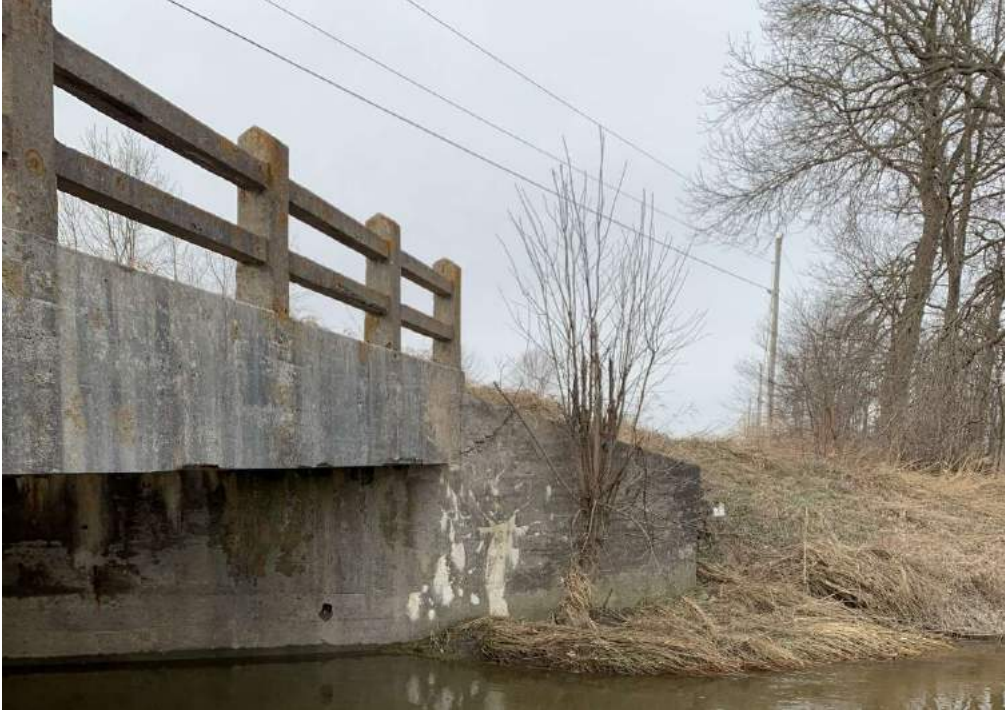
Photo 1-12 - Abutment wall drain and wingwall
