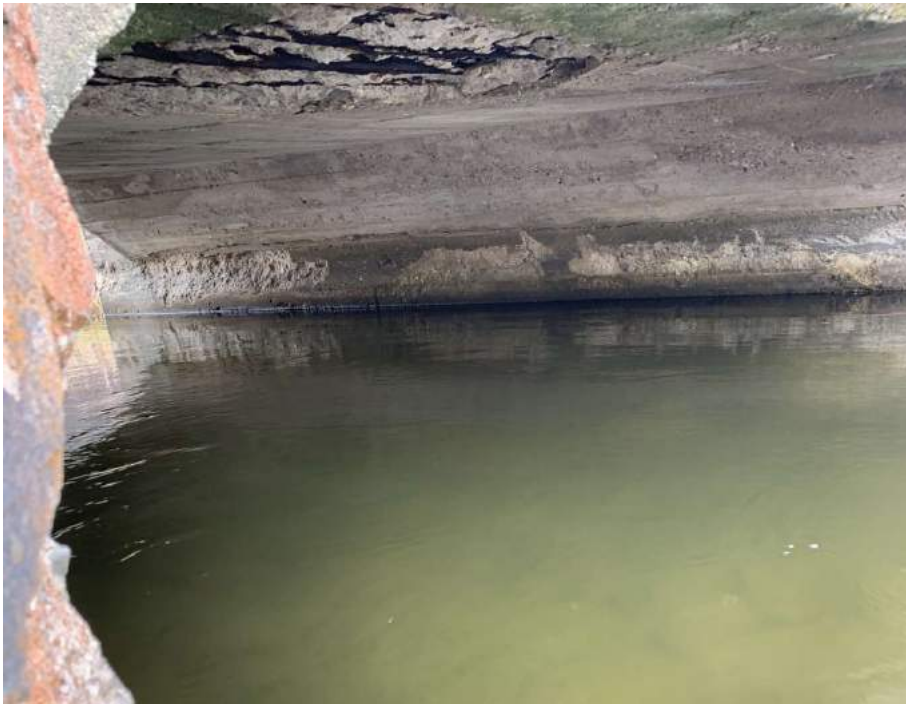
Photo 4-3: View of soffit and abutment wall
