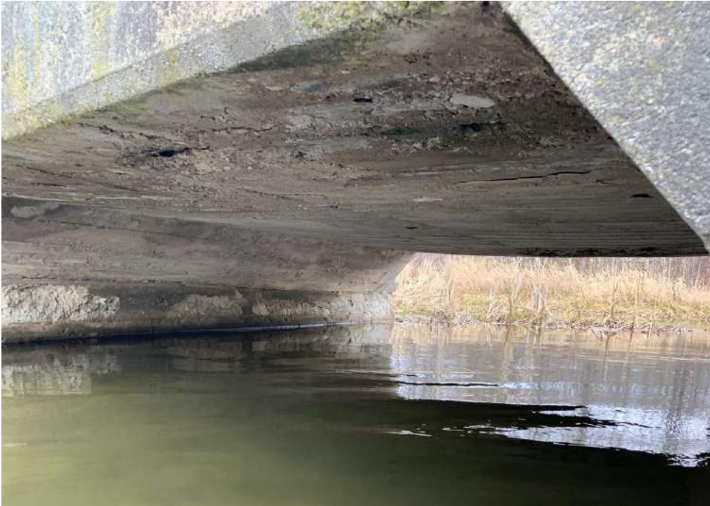
Photo 4-4: View of soffit
