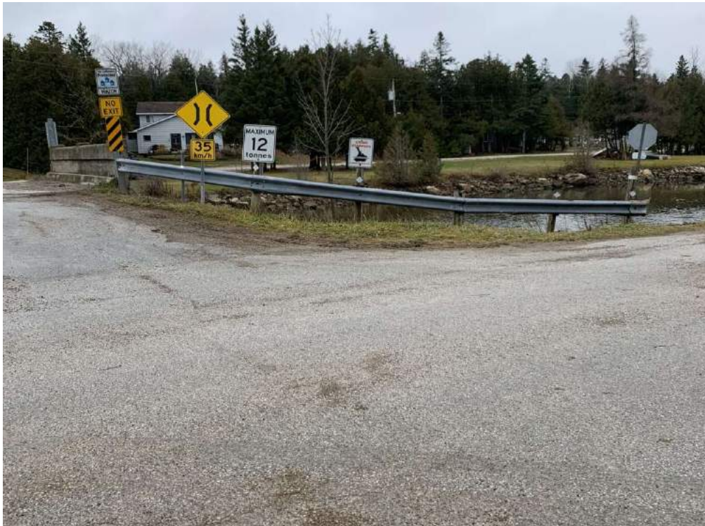
Photo 6-5: View of approach barrier flex beam and wood posts
