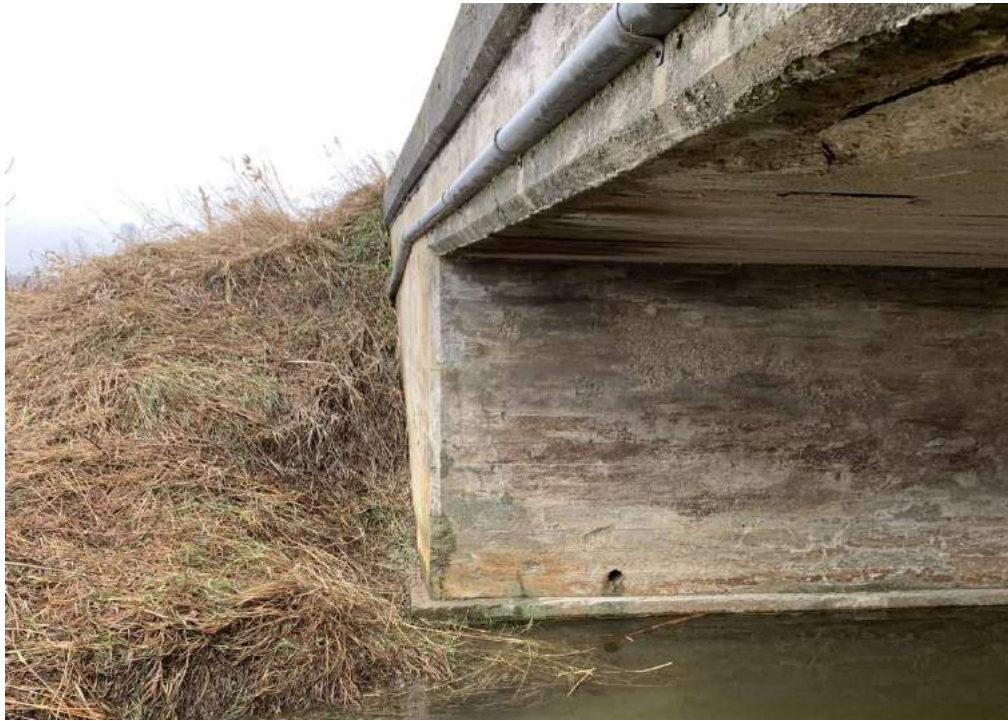
Photo 13-8: View of south abutment wall and exposed footing
