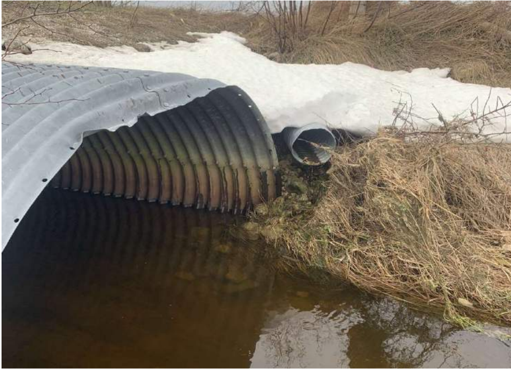
Photo 17-6: View of embankment
