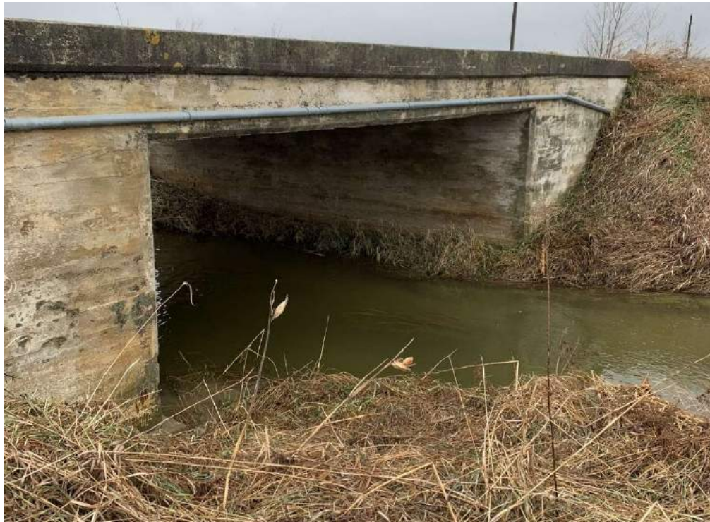
Photo 13-6: View of east structure elevation, exterior soffit and north abutment wall
