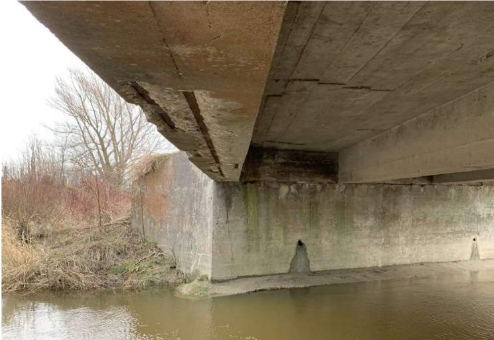
Photo 1-2: South abutment, soffit and exterior girder.
