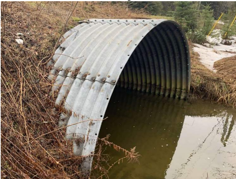
Photo 12-5: View of culvert outlet
