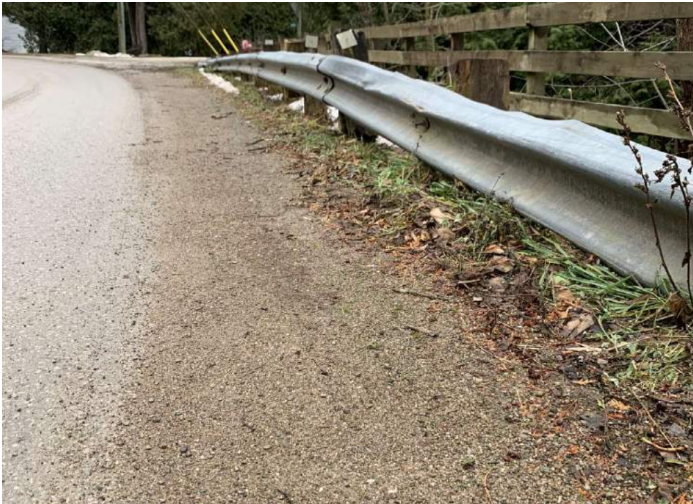
Photo 5-5: Pedestrian (south side only) and structure barrier (typ)
