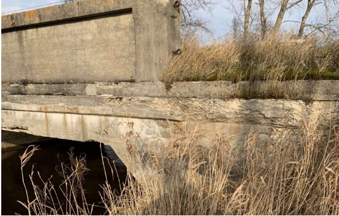
Photo 3-6: East structure elevation, exterior girder and barrier wall
