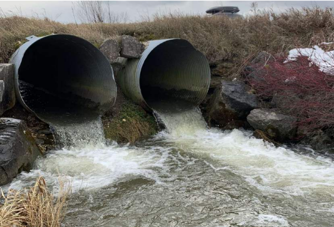
Photo 18-3: View of culvert in elevation and outlet end components
