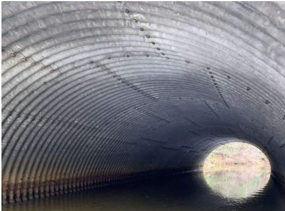
Photo 12-3: View of culvert barrel interior
