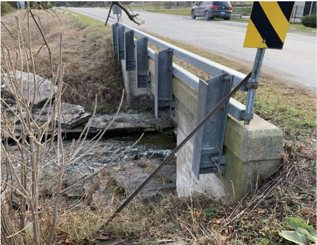
Photo 8-7: View of east structure elevation, wingwalls, exterior soffit and curb
