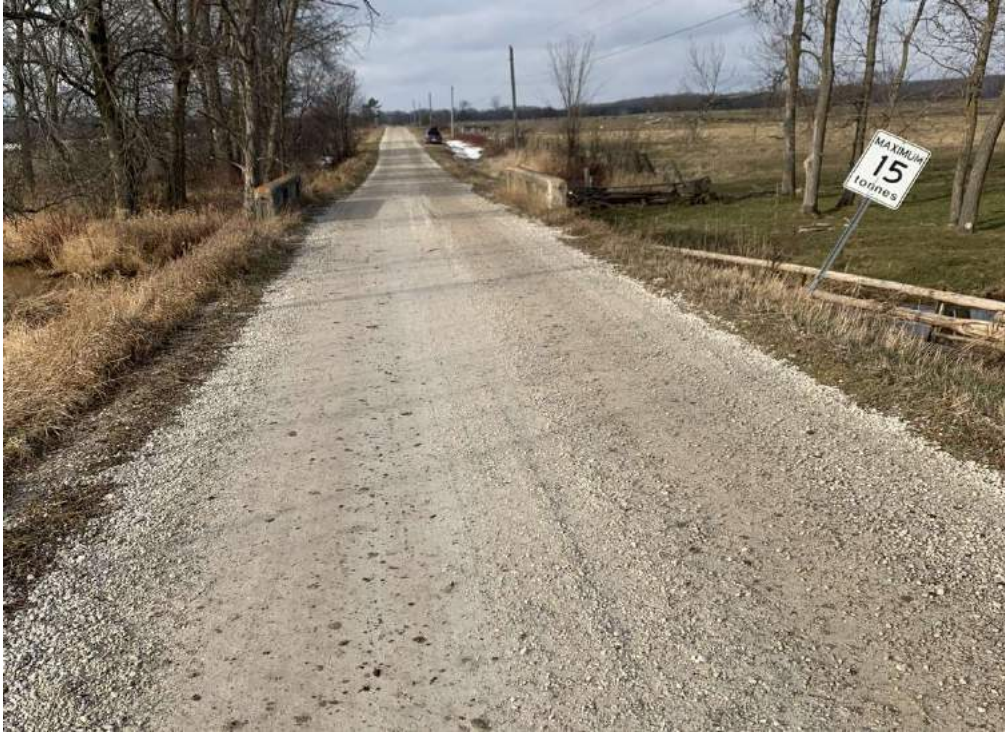
Photo 3-2: View of structure from the south approach
