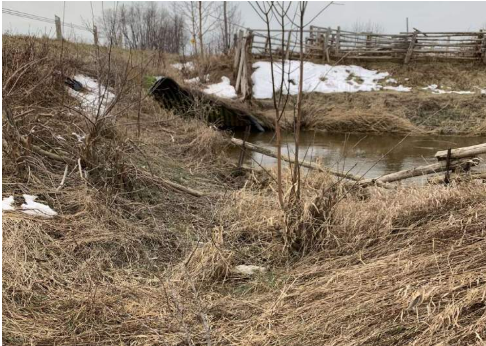
Photo 16-2: View of culvert barrel in elevation (outlet end)
