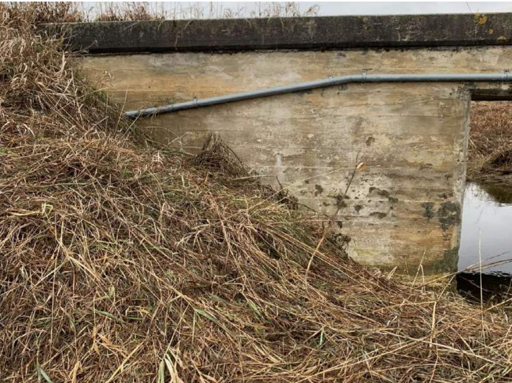
Photo 13-5: Southwest structure wingwall (typical)
