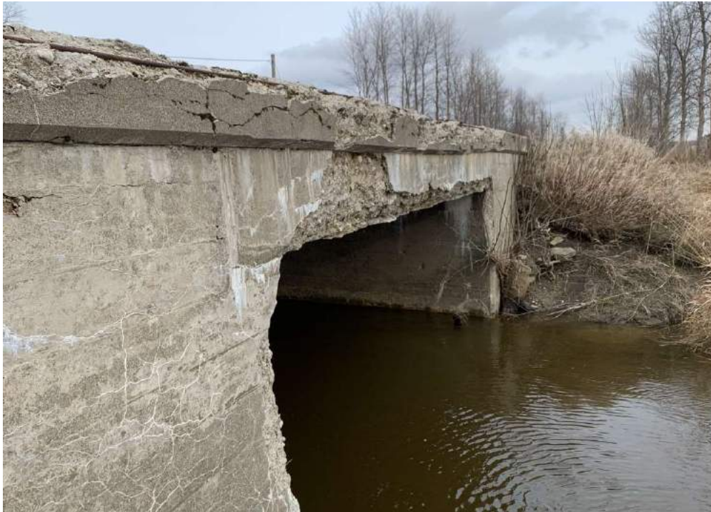
Photo 2-4: West abutment and south exterior soffit
