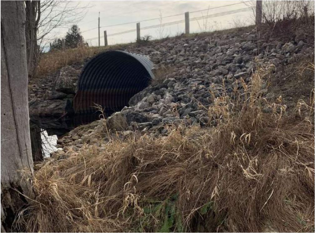
Photo 14-7: View of slope protection
