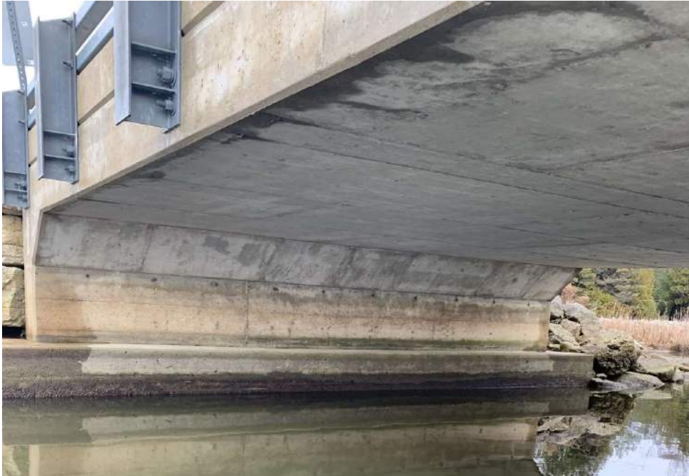
11-6: View of north abutment wall and soffit
