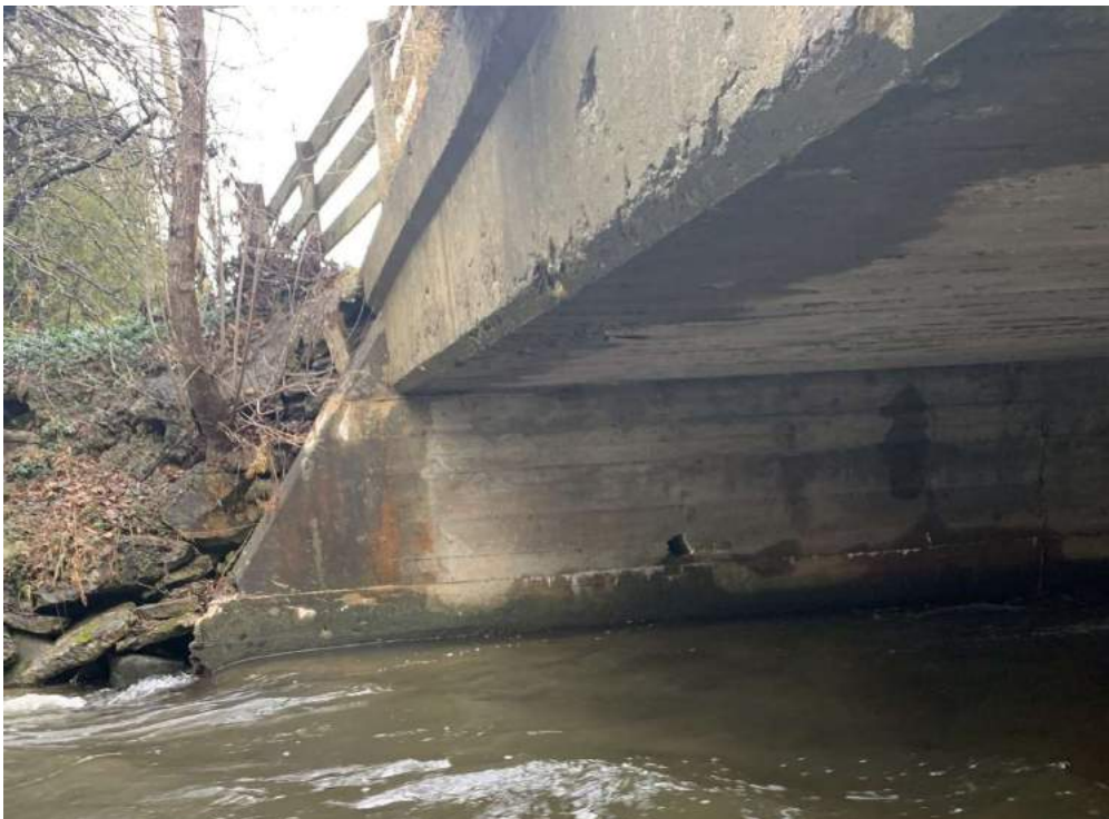
Photo 5-7: View of structure exterior soffit and curb
