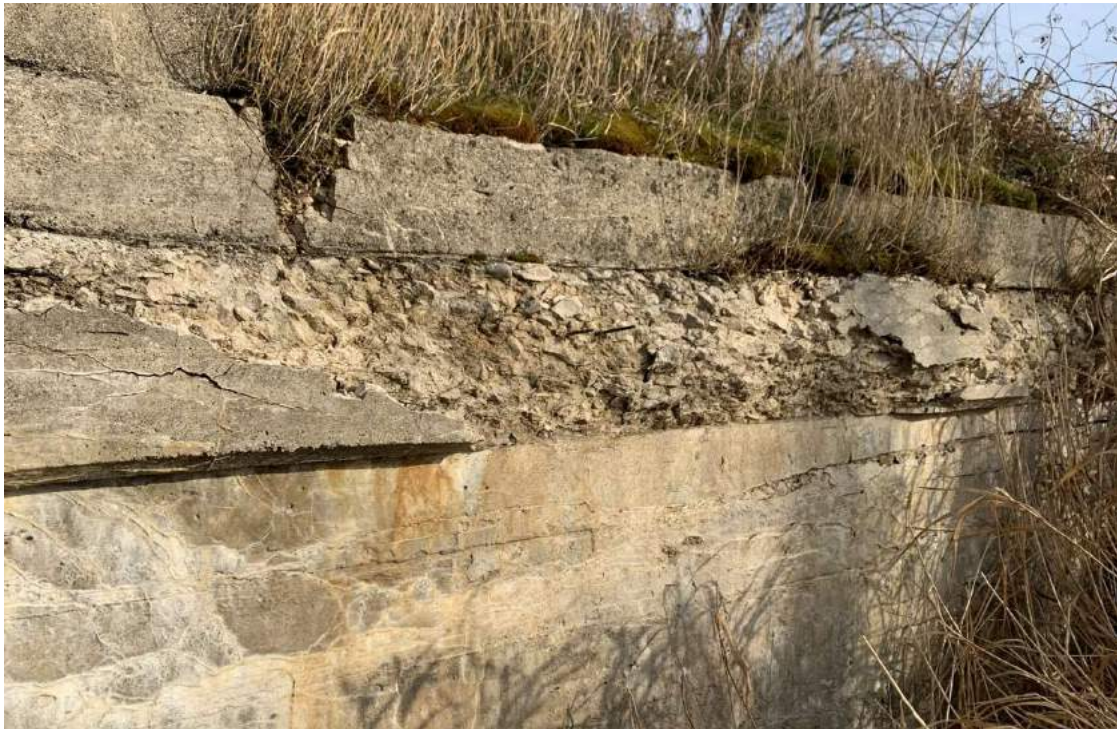
Photo 3-7: Wingwall and exterior curb (typical)
