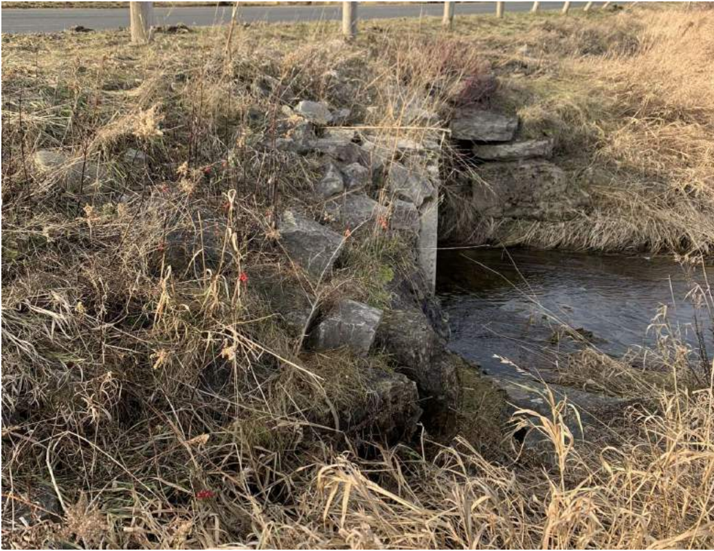
Photo 9-2 - View of structure inlet elevation and embankment
