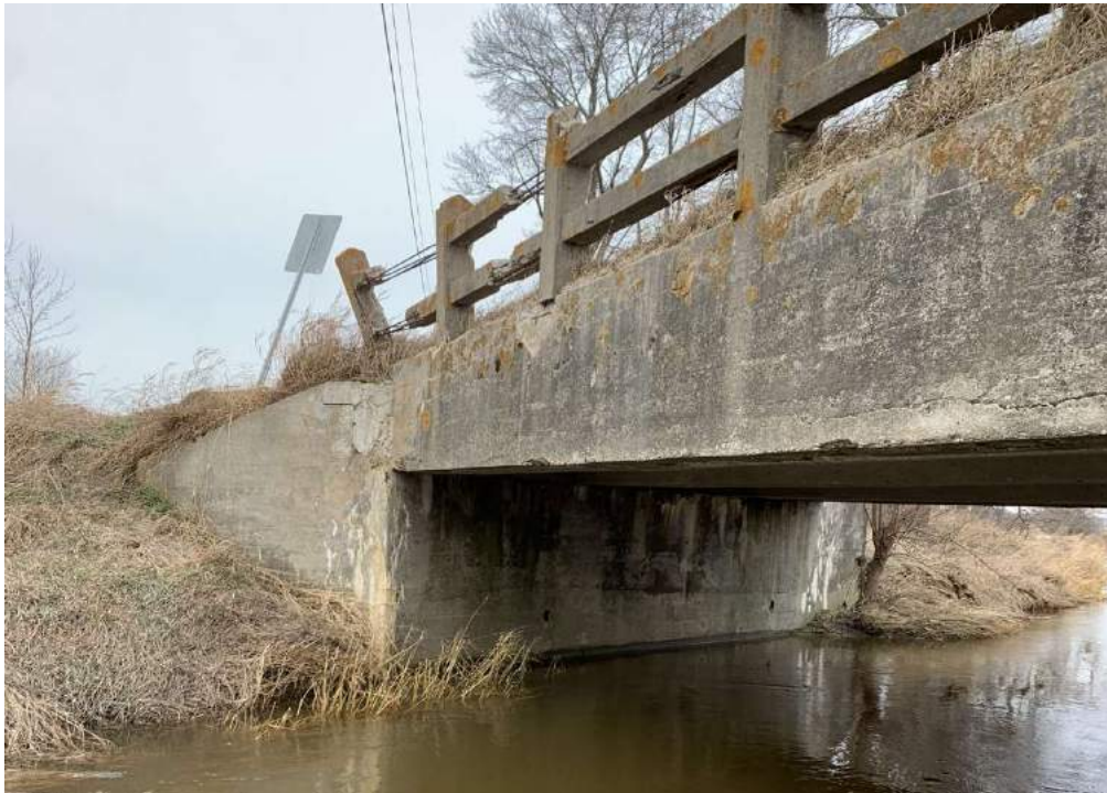
Photo 1-9 - Structure elevation, exterior soffit, curb and barrier
