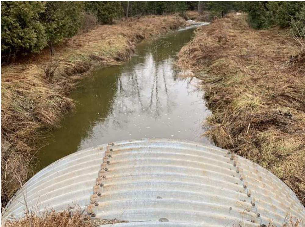
Photo 12-7: View of watercourse upstream
