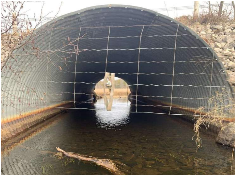
Photo 14-9: View of culvert interior
