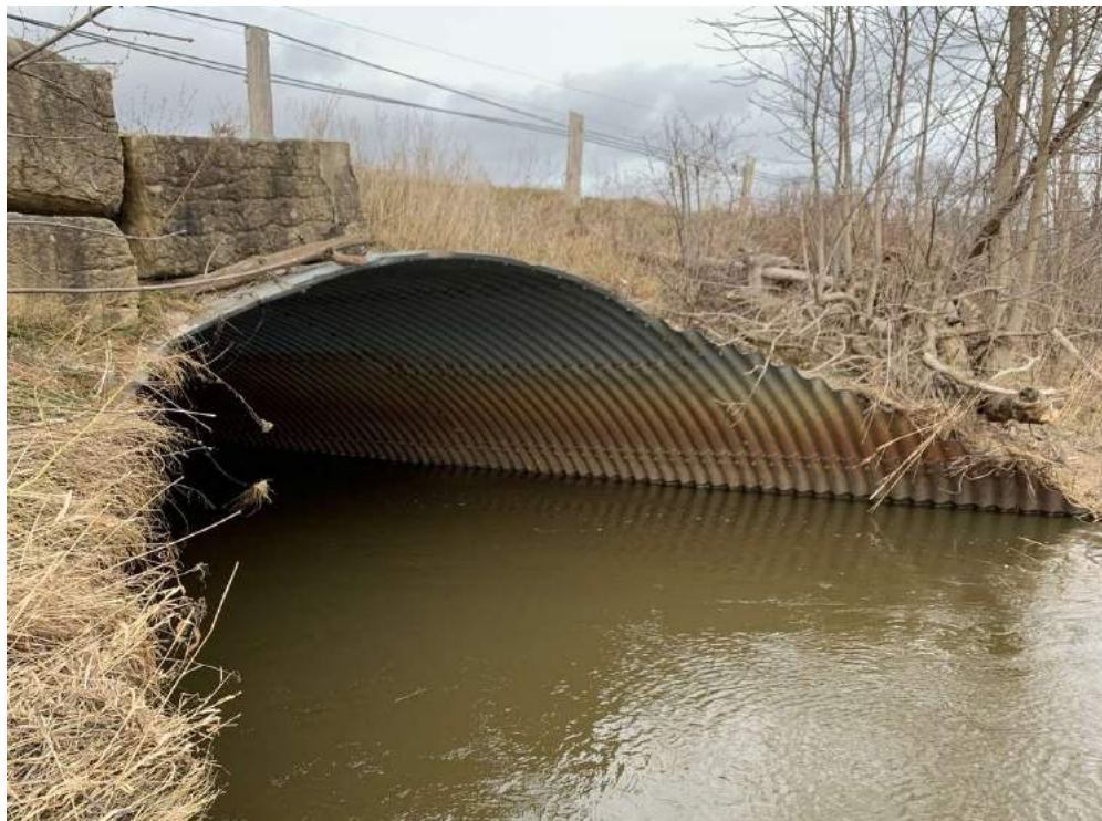
Photo 16-3: View of culvert barrel in elevation (inlet end)
