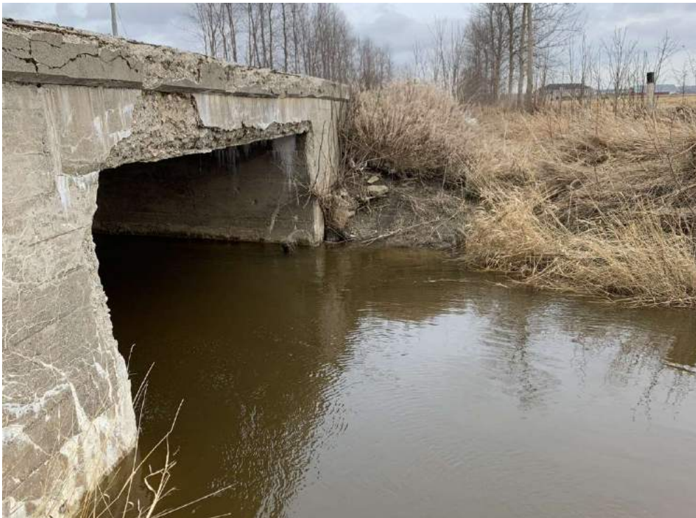
Photo 2-5: Structure elevation, wingwalls, exterior curb and soffit
