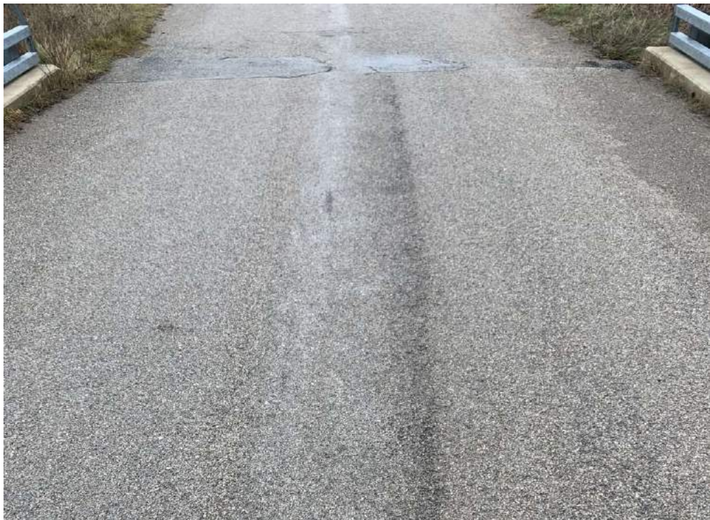
11-11: Structure wearing surface
