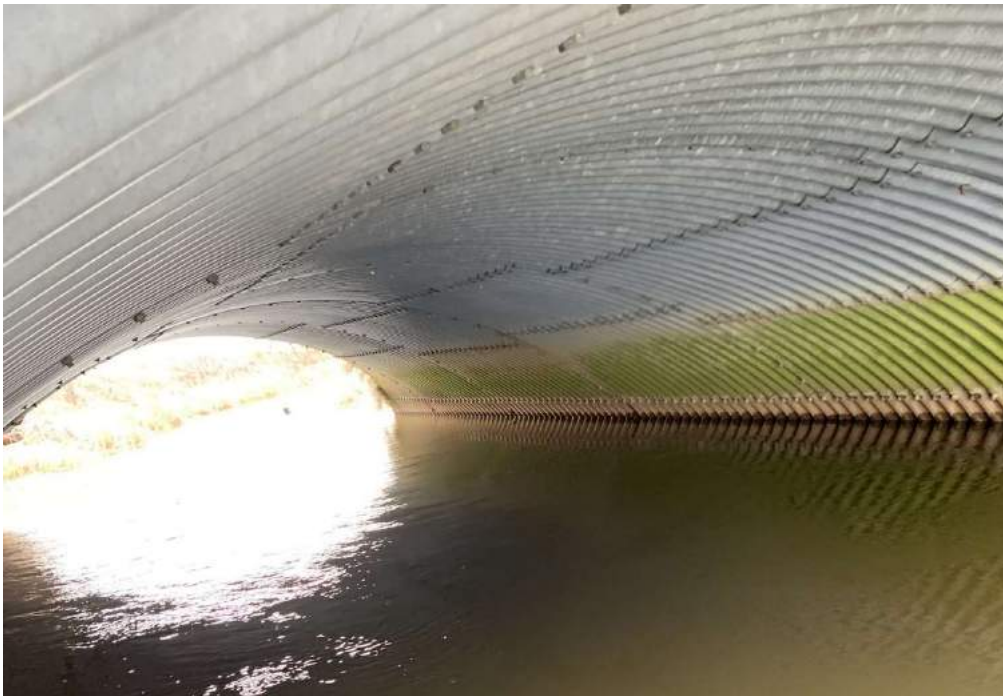
Photo 16-6: Culvert barrel interior
