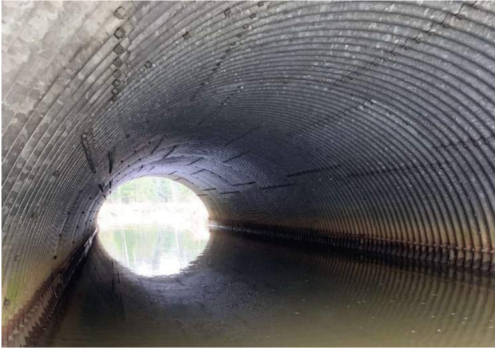
Photo 12-8: View of culvert barrel interior
