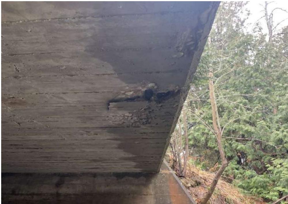
Photo 5-8: View of structure soffit
