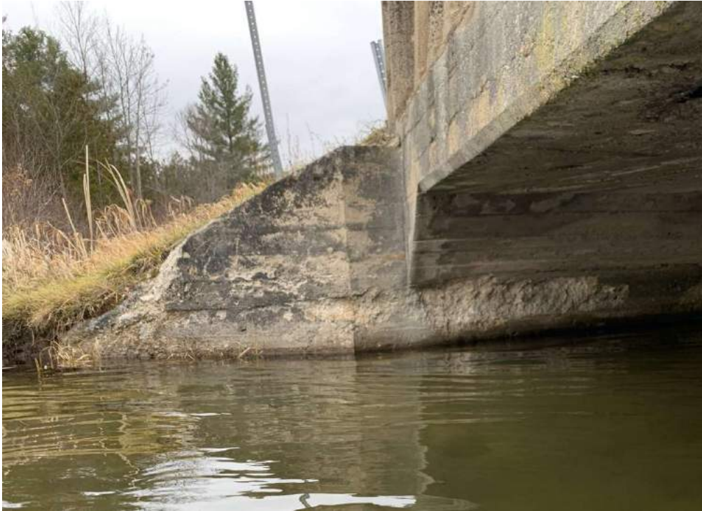
Photo 4-6: View of south abutment wall
