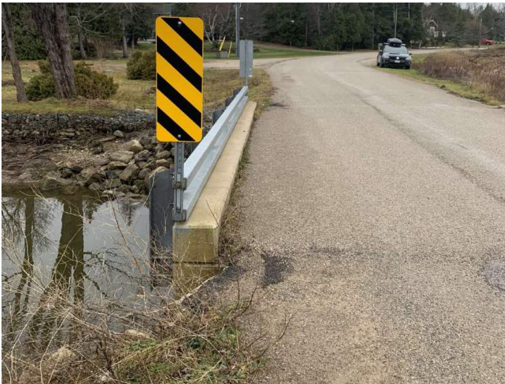
11-7: View of structure wearing surface, barrier protection and end hazard signage
