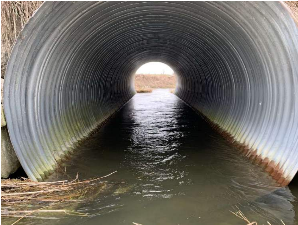
Photo 15-7: View of culvert barrel interior
