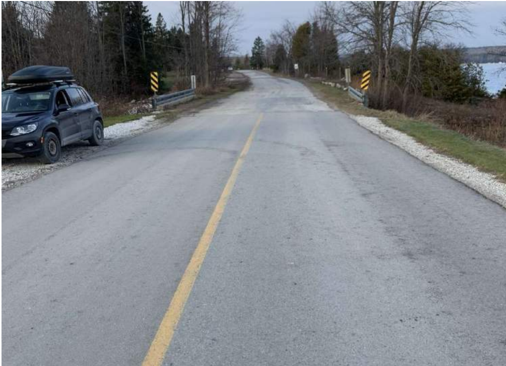
Photo 8-2: View of structure barrier, signage (typ) and encroaching vegetation
