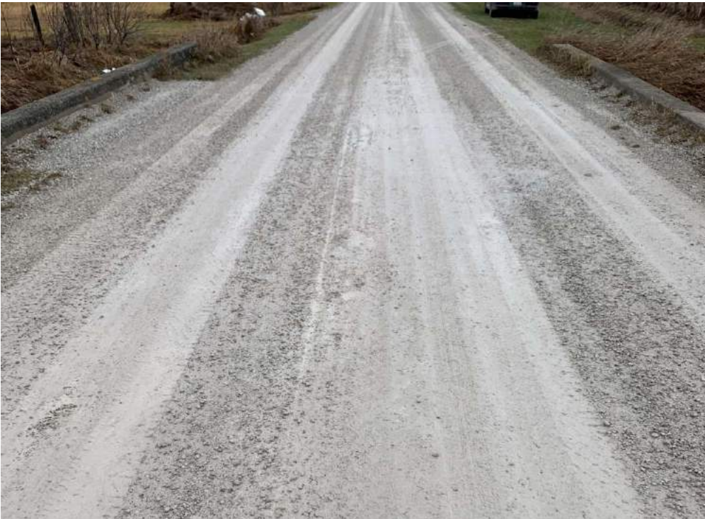
Photo 13-4: Approach and structure wearing surface
