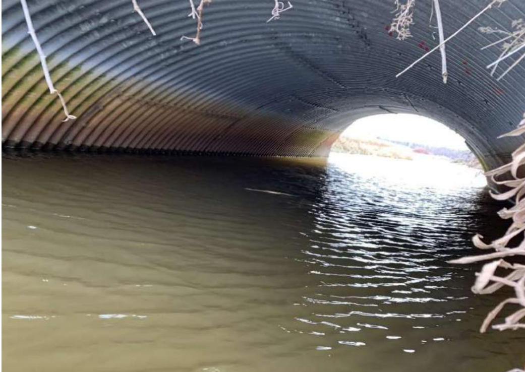
Photo 19-4: View of culvert barrel interior
