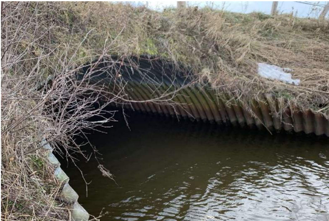
Photo 19-3: View of culvert in elevation and outlet components
