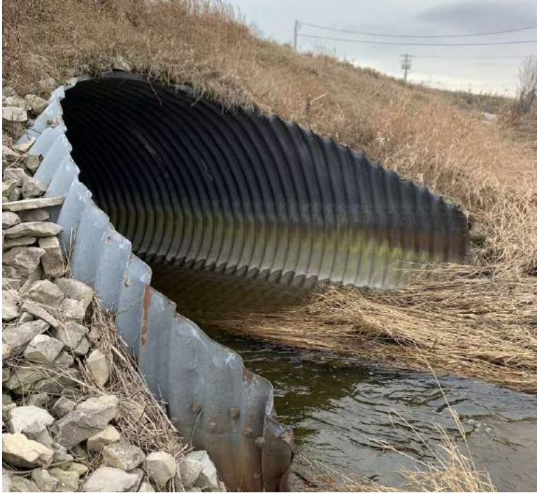
Photo 10-4: View of culvert barrel in elevation
