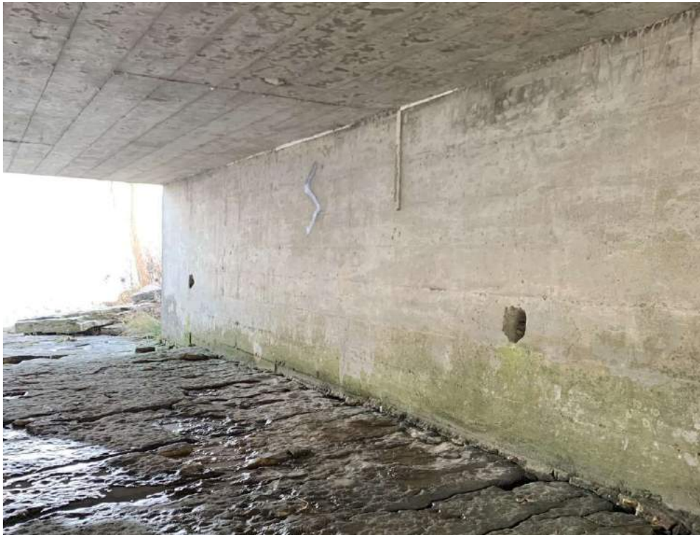
Photo 8-9: View of south abutment wall and soffit
