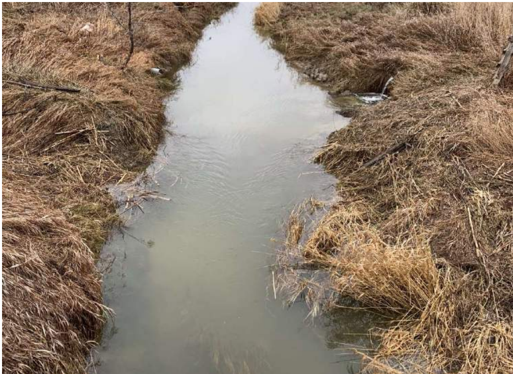
Photo 13-9: View of watercourse upstream
