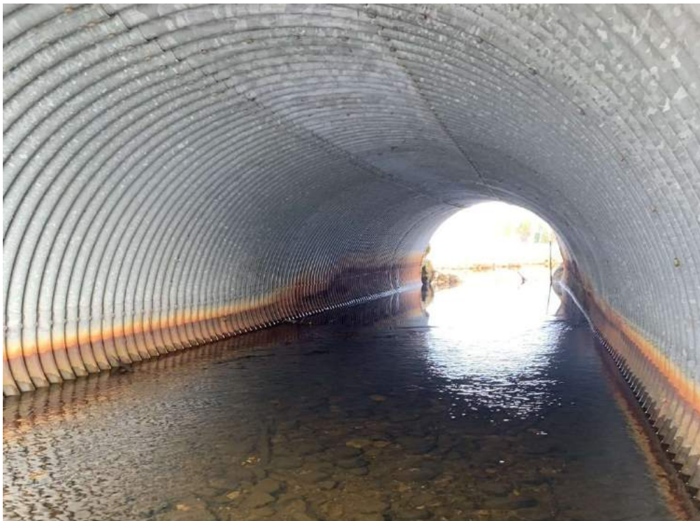
Photo 14-5: View of culvert barrel interior, obvert
