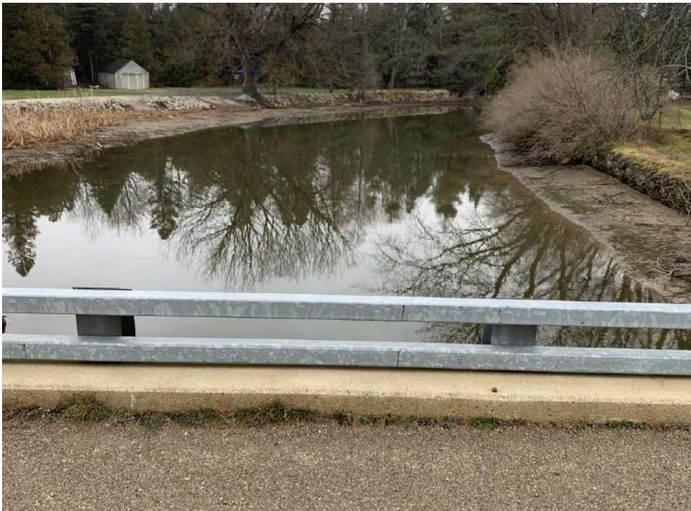
11-7: View of watercourse upstream
