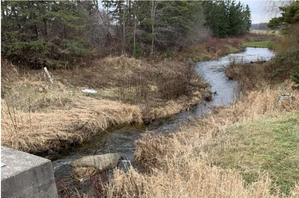
Photo 7-2: View of watercourse upstream and upstream culvert end
