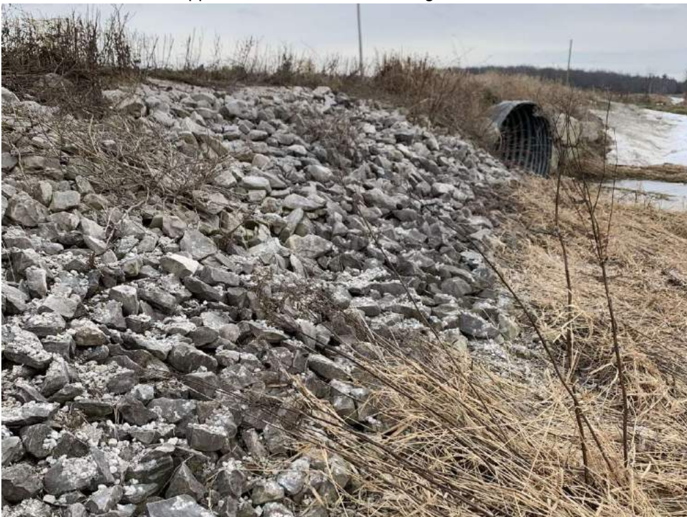
Photo 15-3: Rock protection at inlet end
