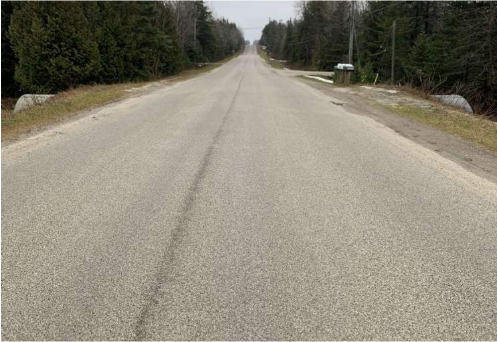
Photo 12-4: View of surface treatment wearing surface
