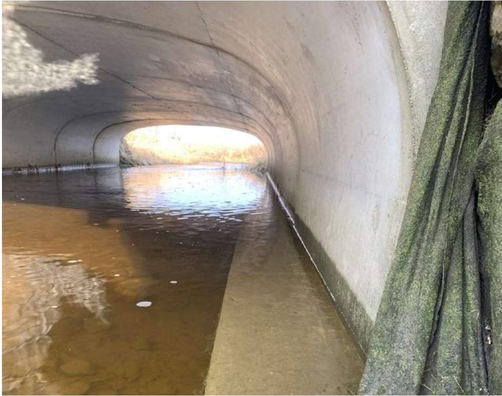
Photo 9-4 - View of pipe arch soffit and walls
