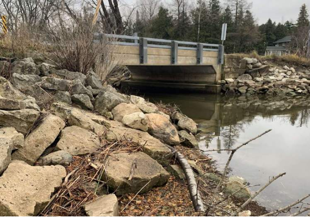
Photo 11-2: View of east structure elevation, exterior soffit, barrier and embankments
