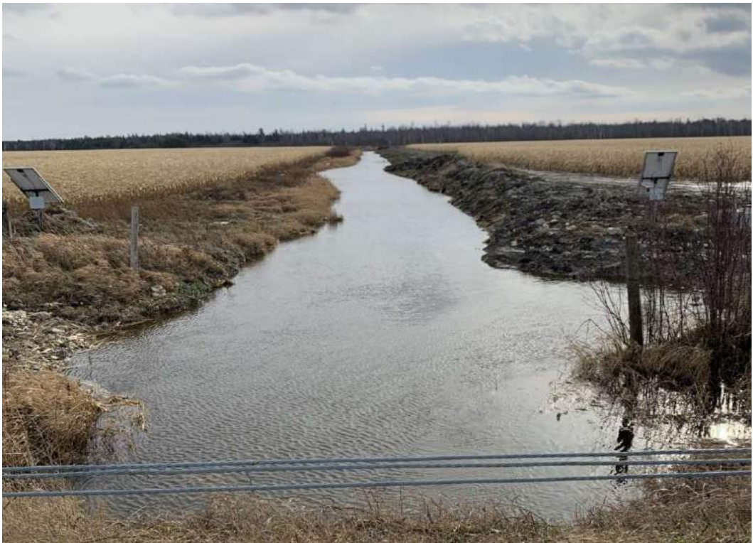
Photo 19-9: View of structure downstream
