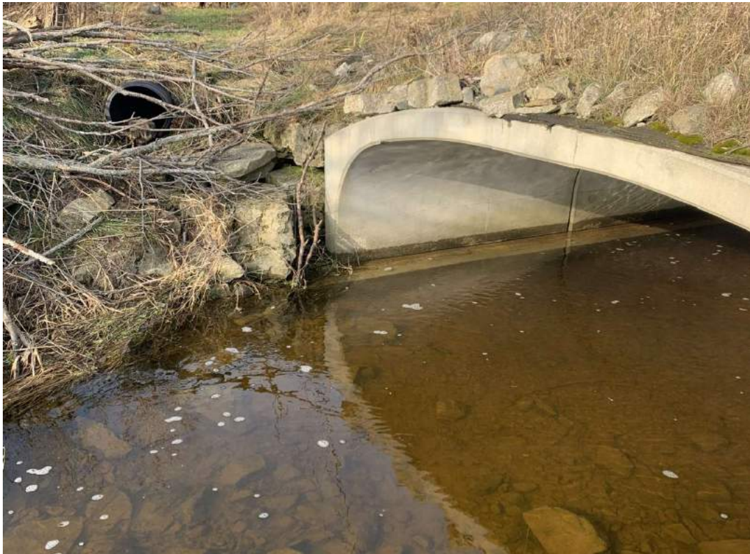
Photo 9-3 - View of structure outlet elevation and embankments
