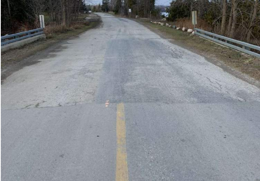
Photo 8-6: View of structure approach and deck wearing surface
