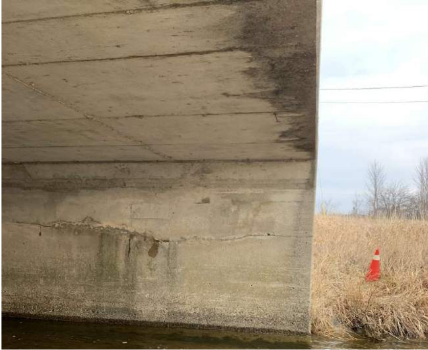
Photo 7-6: View of soffit and abutment walls
