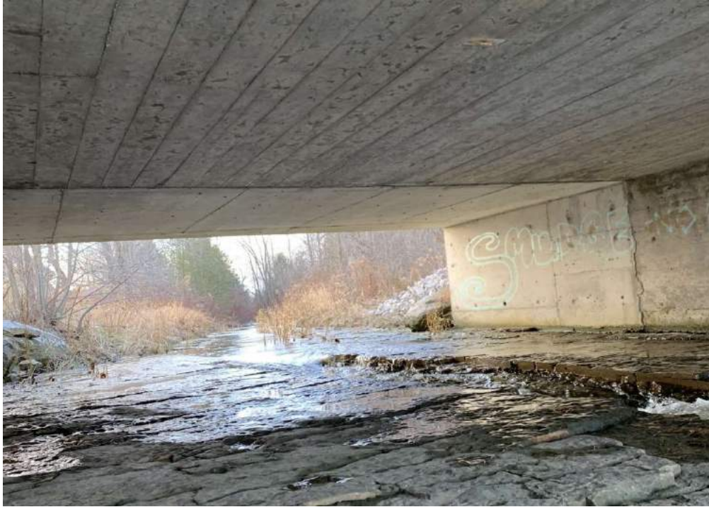
Photo 8-8: View of north abutment wall and bedrock streambed
