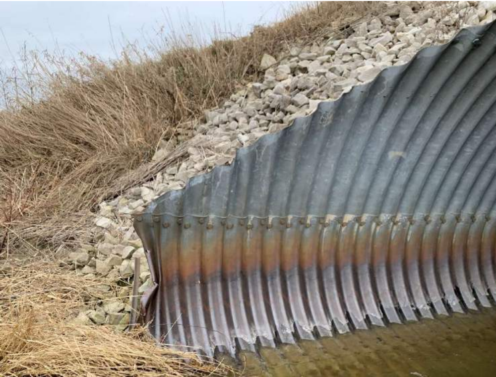
Photo 10-7: View of embankment and culvert inlet interior
