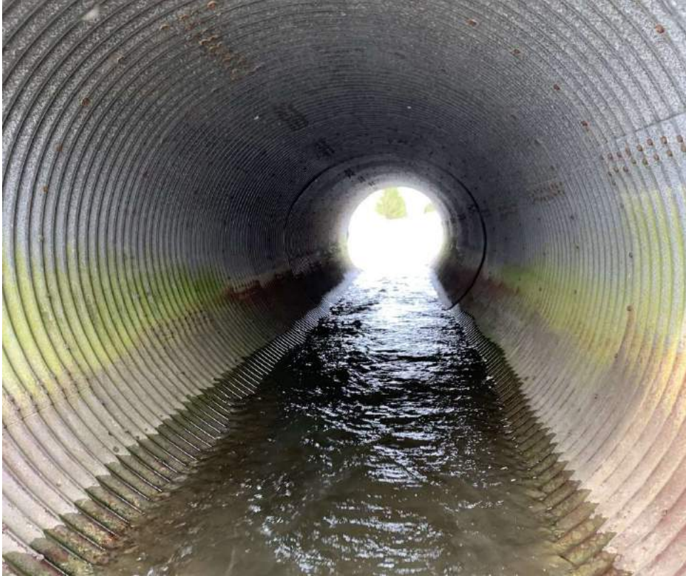
Photo 18-8: View of east culvert barrel interior
