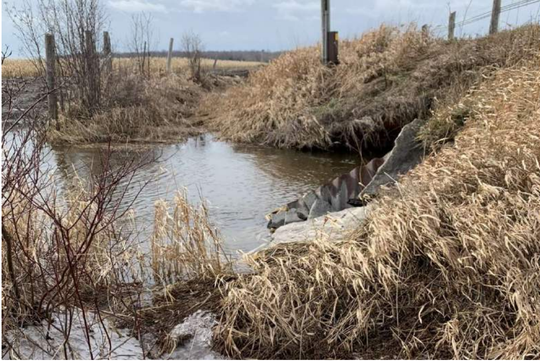
Photo 19-2: View of culvert in elevation and inlet components
