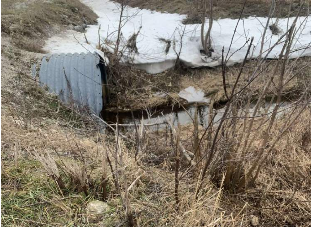
Photo 17-5: View of culvert in elevation and inlet components
