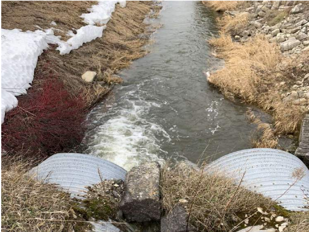
Photo 18-5: View of watercourse downstream and outlet culvert ends
