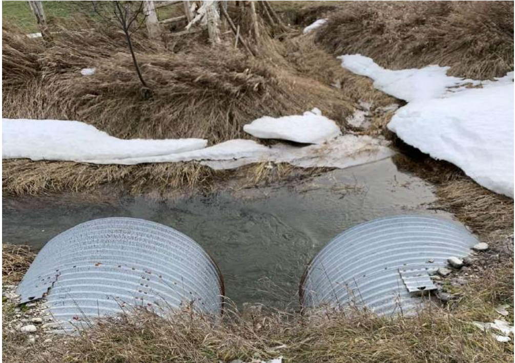
Photo 18-4: View of watercourse upstream and inlet ends
