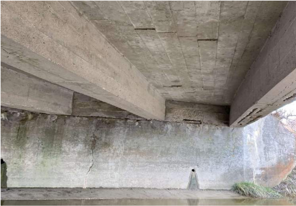
Photo 1-4: South abutment wall, soffit and girders
