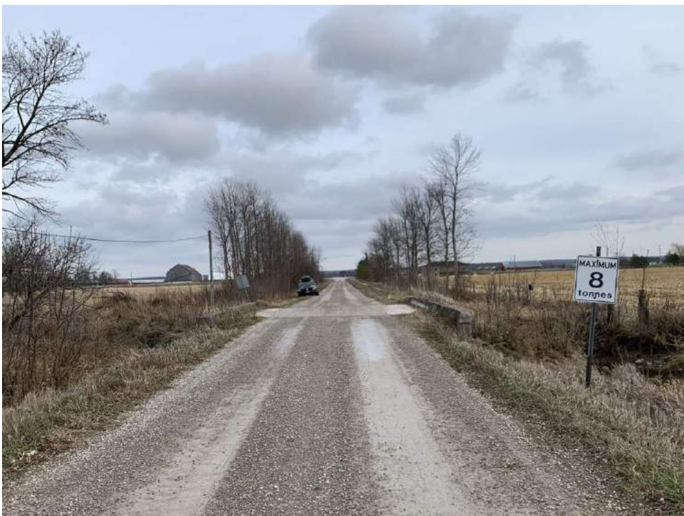
Photo 2-9: Load limit posting
