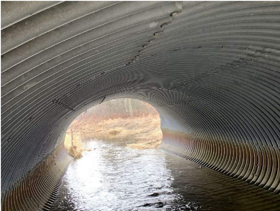
Photo 10-5: View of interior culvert barrel
