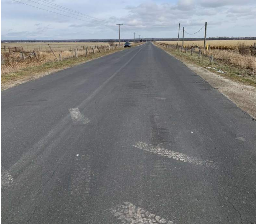
Photo 19-10: View of structure and approach wearing surface
