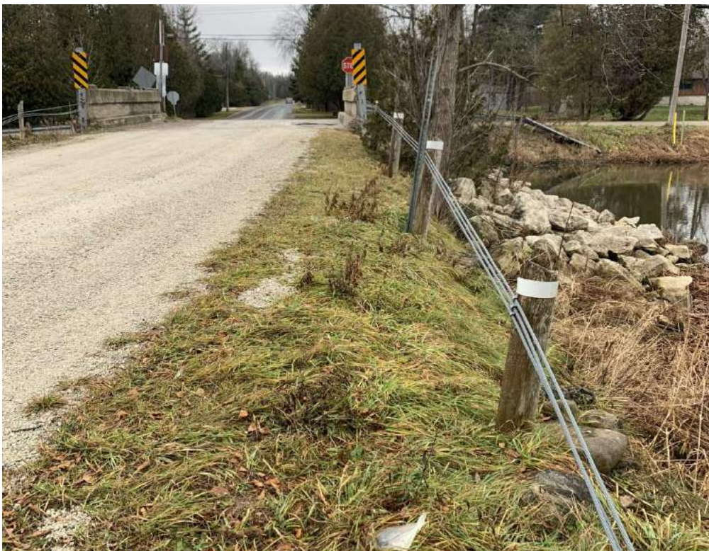
Photo 6-3: View of structure from south approach
