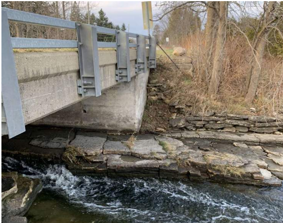
Photo 8-11: View of structure elevation, exterior barrier protection, curb and soffit
