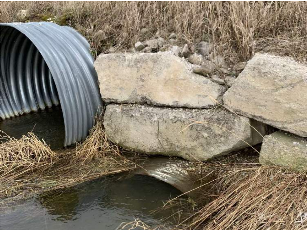
Photo 15-5: View of east culvert end
