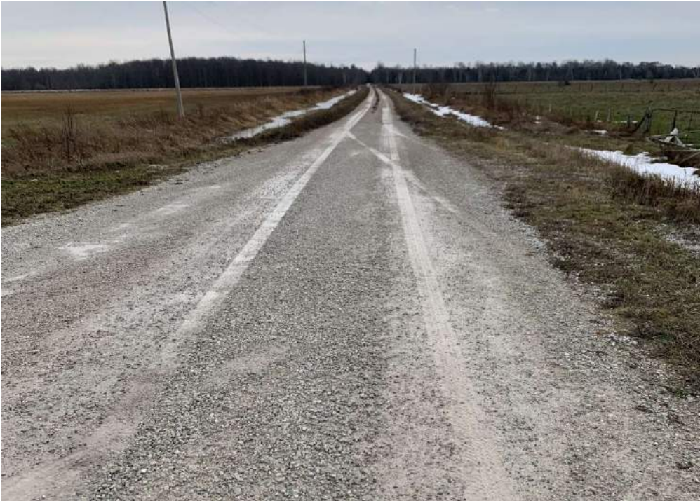
Photo 15-2: View of approach and structure wearing surface
