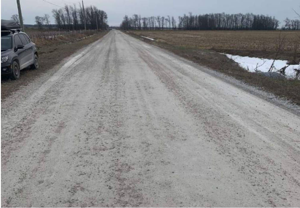
Photo 17-2: View of structure and approach wearing surface
