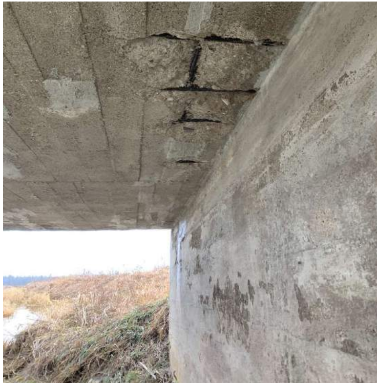
Photo 13-7: View of structure soffit and north abutment wall
