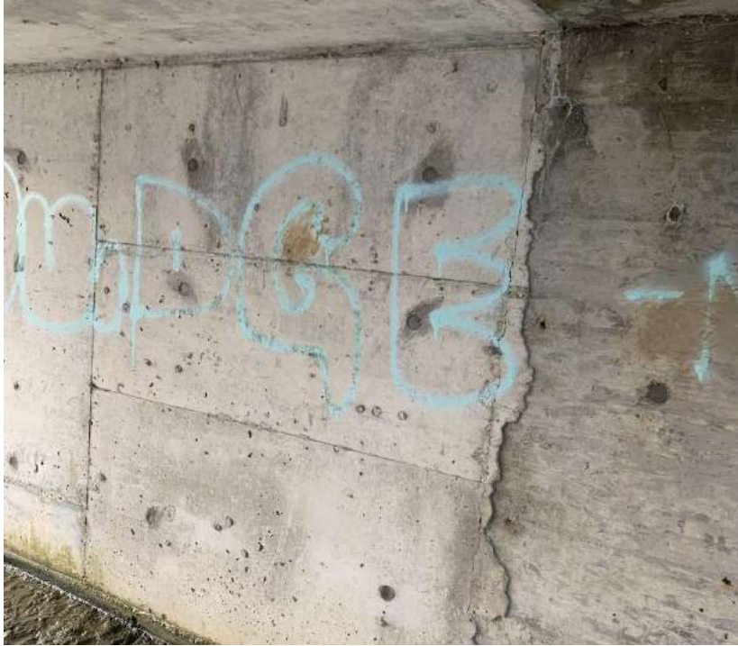
Photo 8-12: View of abutment wall
