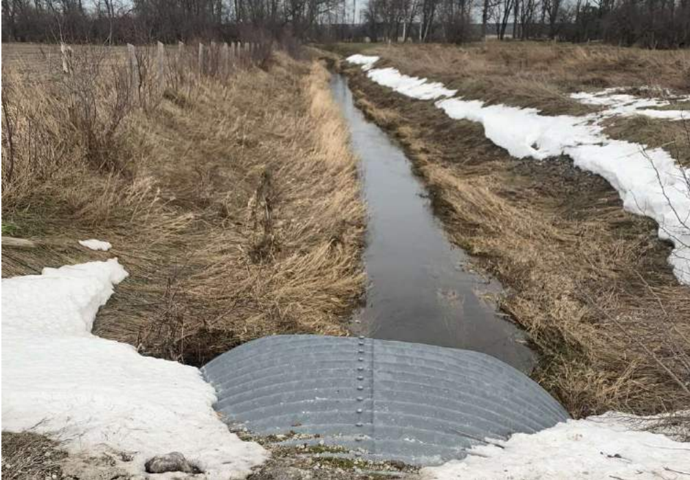
Photo 17-4: View of watercourse downstream and outlet culvert end
