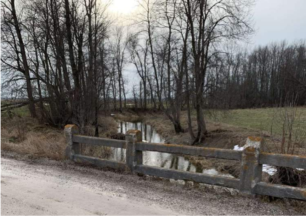
Photo 1-10 - View of watercourse upstream
