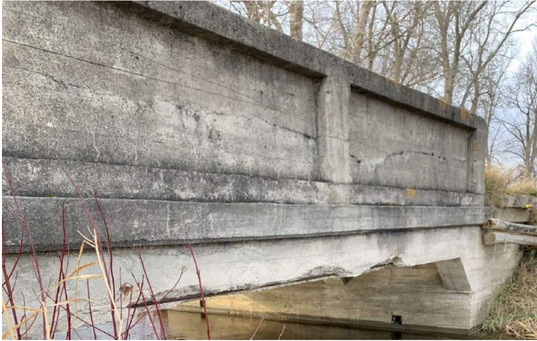
Photo 3-10: View of west structure elevation, exterior girder and barrier wall
