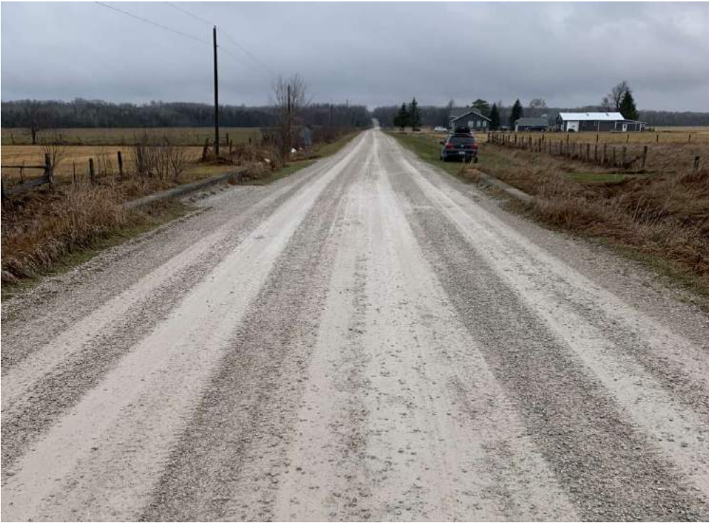
Photo 13-2: View of structure from the south approach
