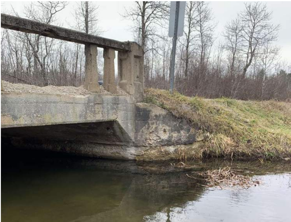
Photo 4-7: View of west structure elevation, exterior soffit, curb and barrier
