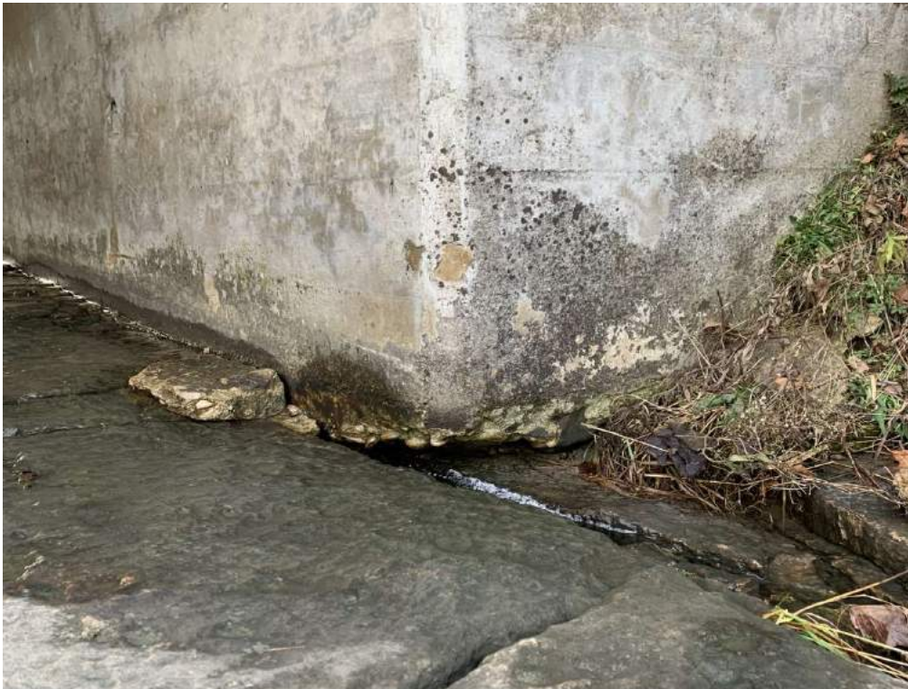
Photo 8-13: View of wingwall
