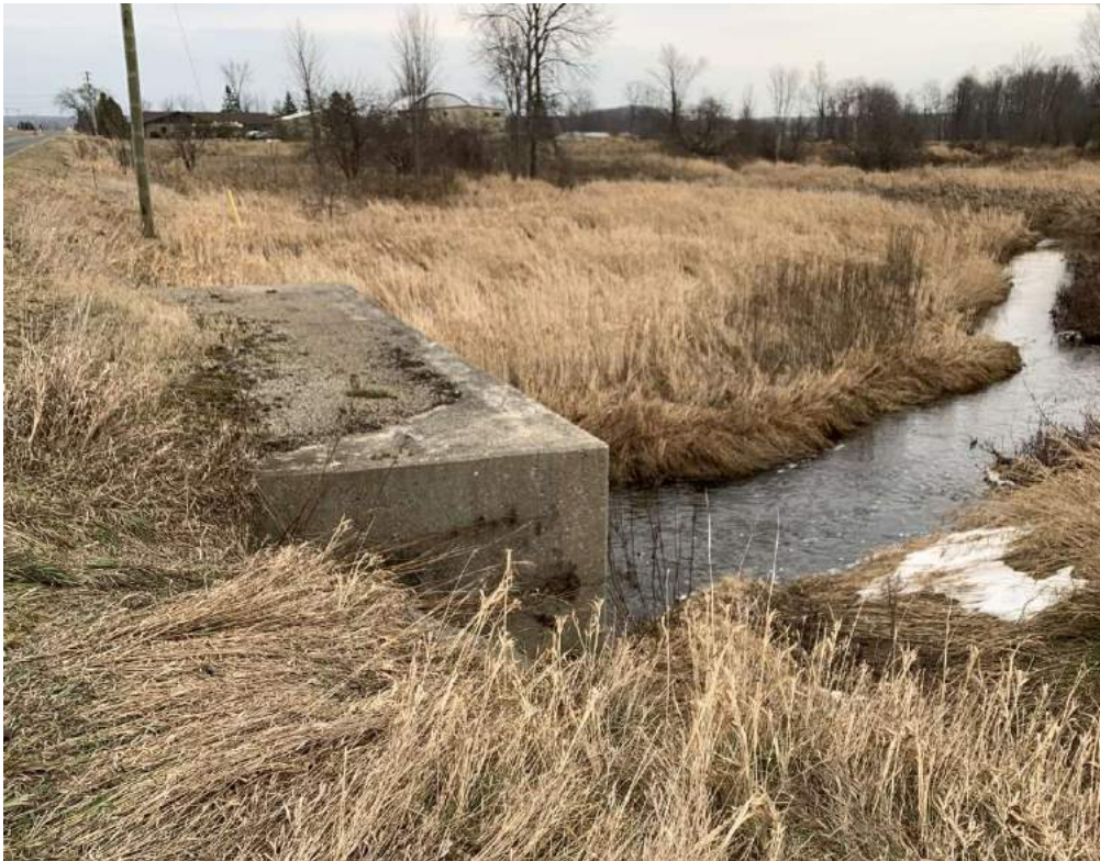
Photo 7-3: View of watercourse downstream and downstream culvert end
