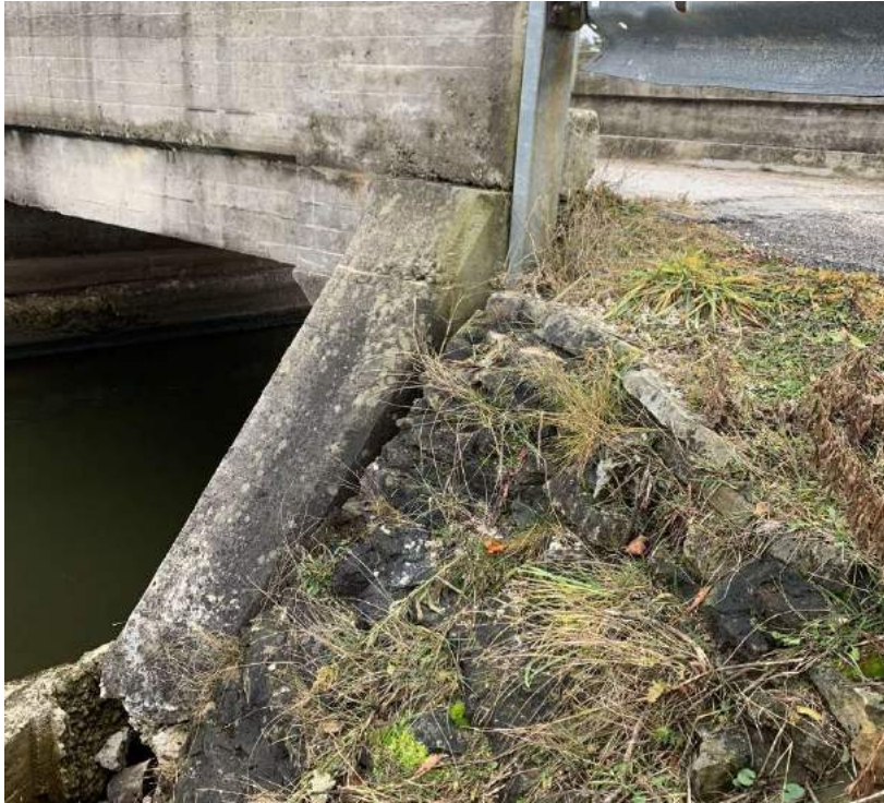
Photo 6-6: View of west structure elevation, wingwalls, exterior curb and parapet wall
