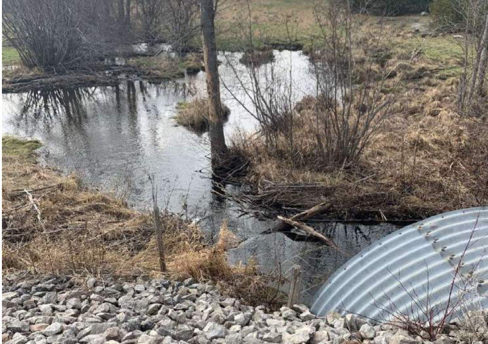
Photo 14-4: View of watercourse upstream
