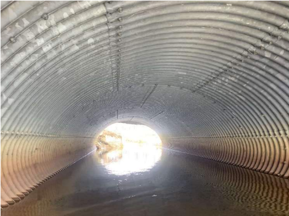
Photo 17-7: View of culvert barrel interior
