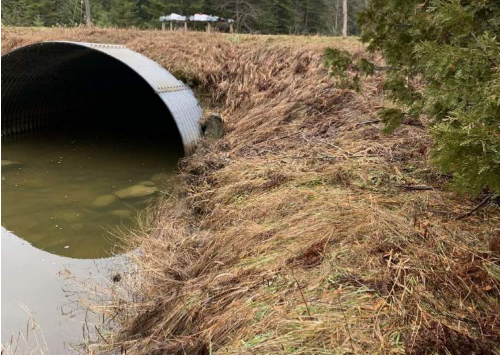
Photo 12-2: View of culvert inlet in elevation (north perspective)
