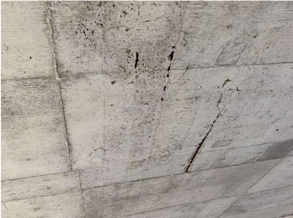
Photo 7-7: View of soffit
