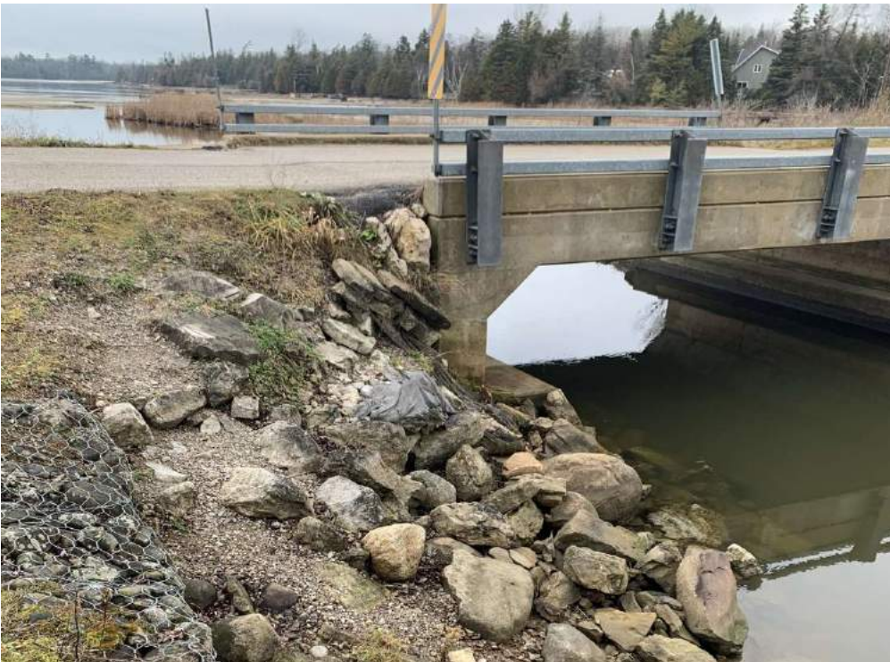
Photo 11-3: View of exterior barrier protection, soffit and wingwalls
