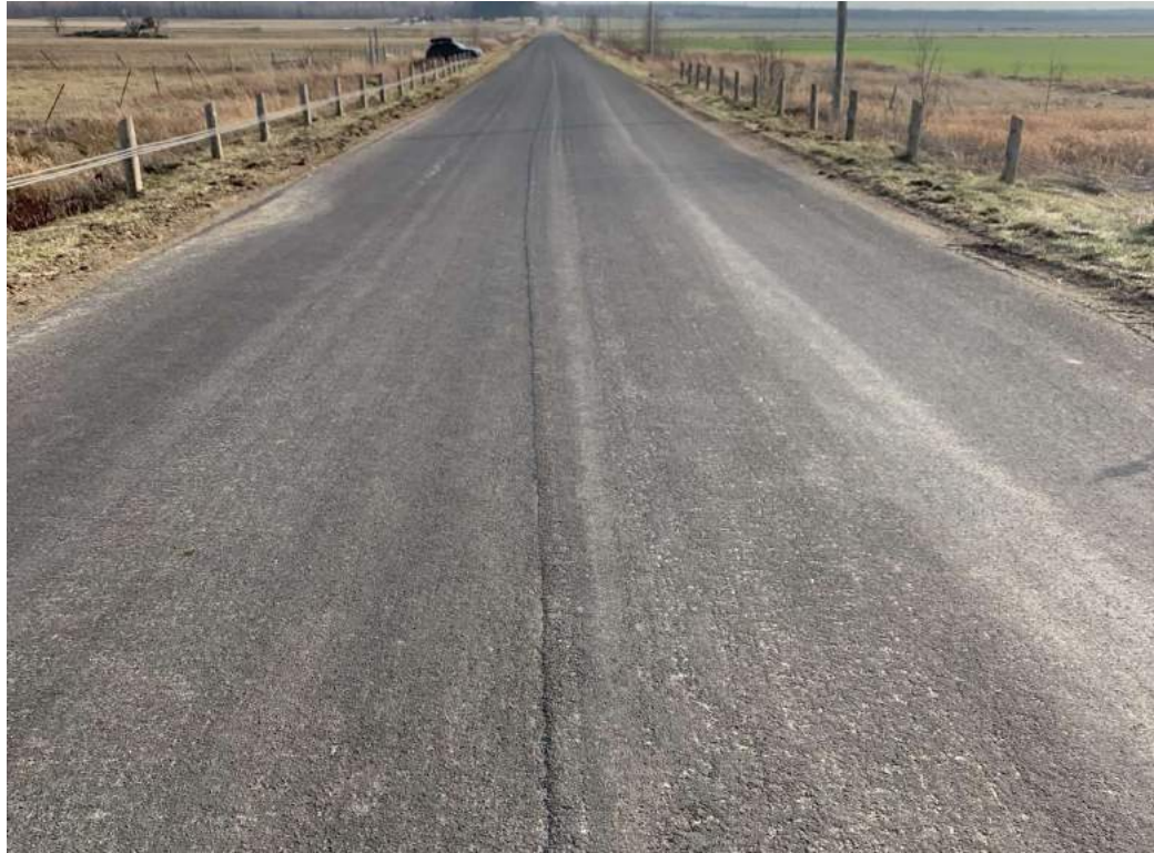
Photo 9-9 - View of structure wearing surface from approaching perspective
