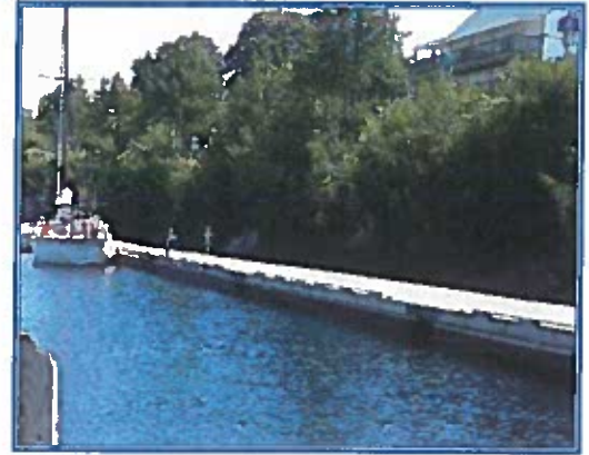
Figure 4.4: Wooden jetty, looking east from the southern steel dock
