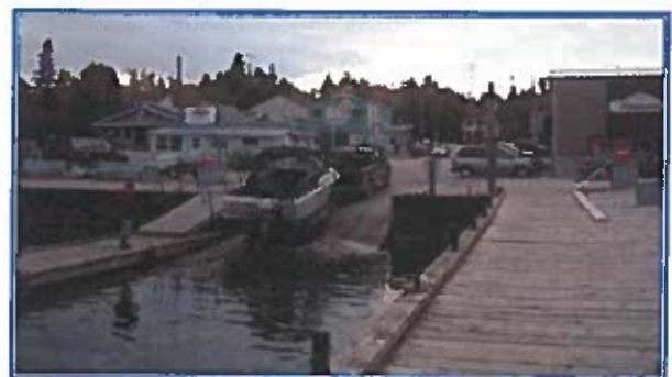
Figure 4.2: Boat launch ramp in the west wall, looking west from the north wharf
