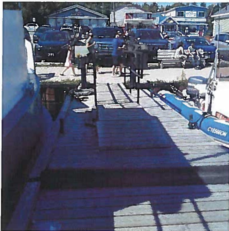
Figure 6: Pedestrian Access Ramp from West Wall to Steel Dock 3-4
