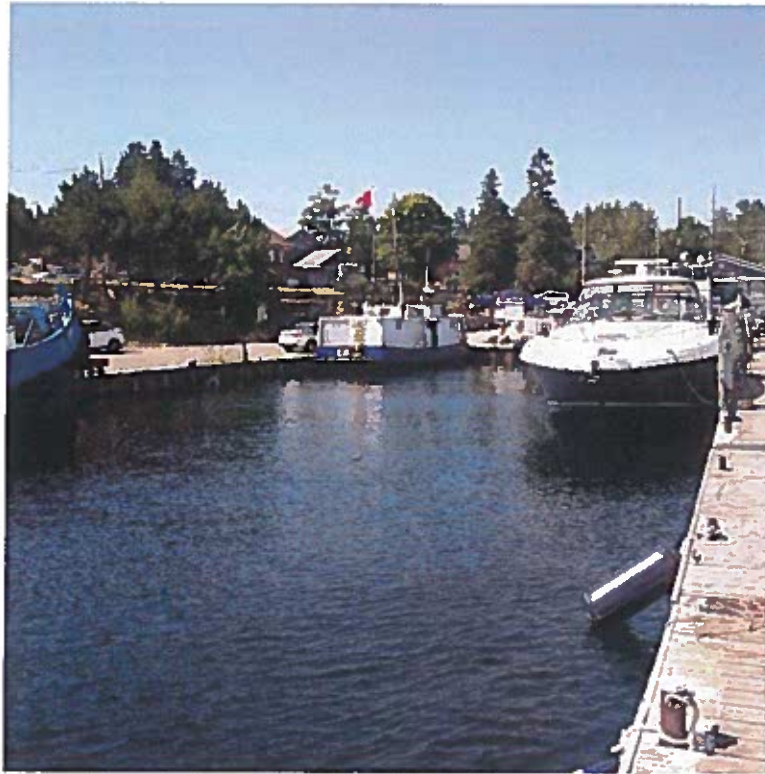
Figure 5: Steel Dock 3-4 and South Wharf, Looking West
